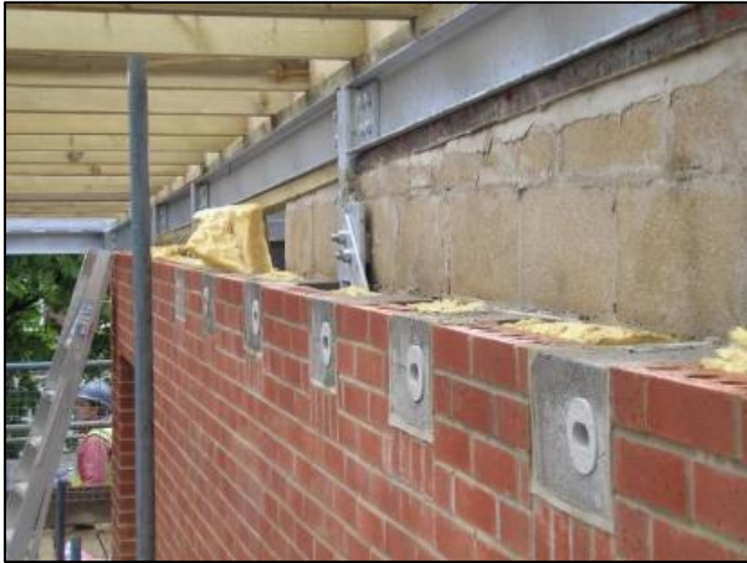
Figure 26: Swift Bricks installed during build phase in Nothing Hill London.
