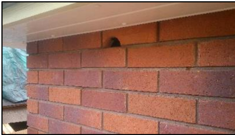
Figure 27: A Swift Brick installed in a newly erected redbrick wall. Photo: www.birdbrickhouses.co.uk
